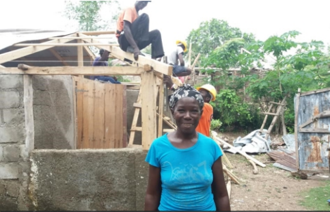
Henriette received one of 5,000 BBS e-vouchers to pay to have the roof of her house rebuilt.
