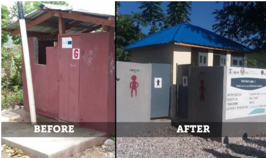
BBS rehabilitated 16 sanitation facilities, reconstructing foundations and walls as needed and installing new fixtures and hand washing stations.
